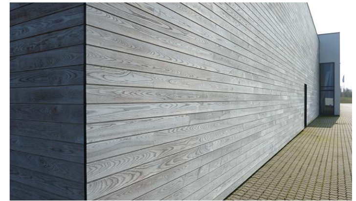
Uncoiled Thermory Benchmark thermo-ash one year after installation Denmark
