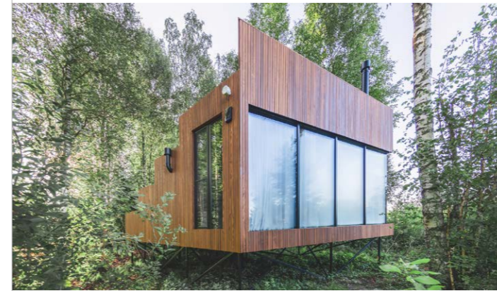
Thermory Benchmark thermo-ash cladding few months after installation. Maida Nature Resort in Estonia Photography Elvo Jakobson
