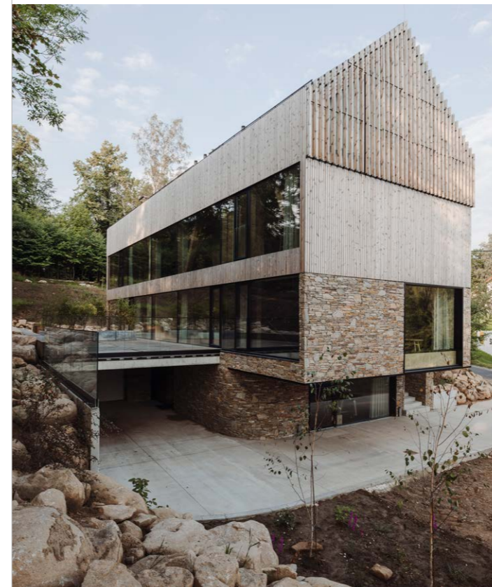
Uncoiled Benchmark thermo-pine cladding and roofing one year after installation. Apartments in Poland Photo and distribution: Komplex Market
