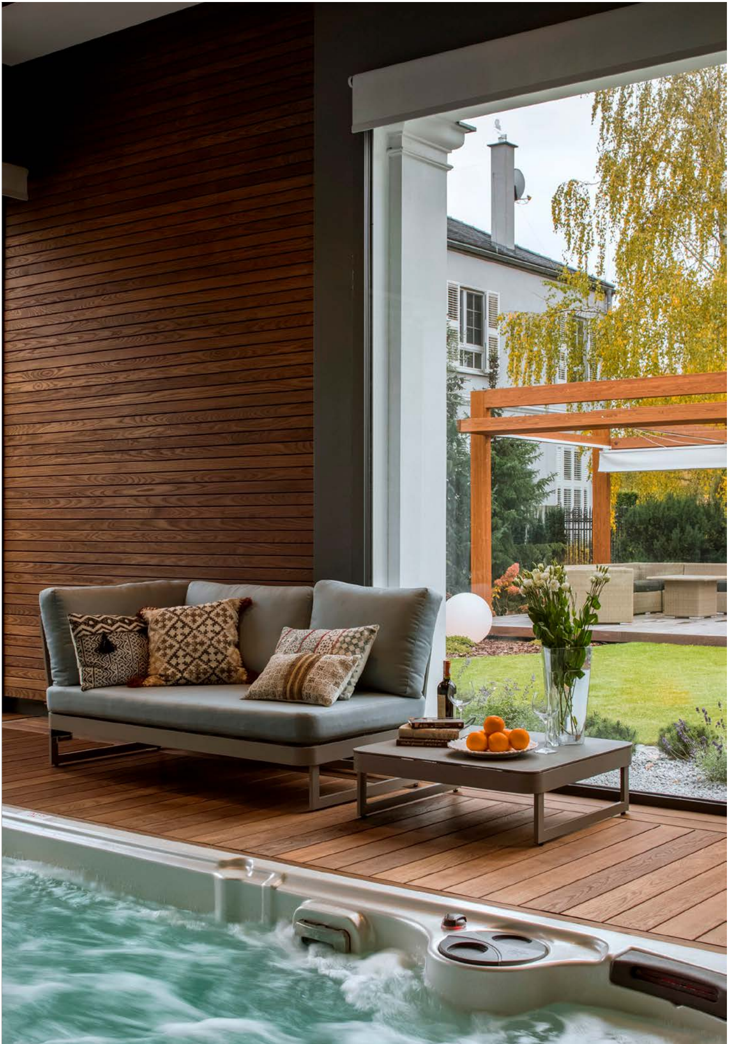
Thermo-ash C7J wall paneling, thermo-ash D4sg2 decking. Photo: Yassen Hristov
